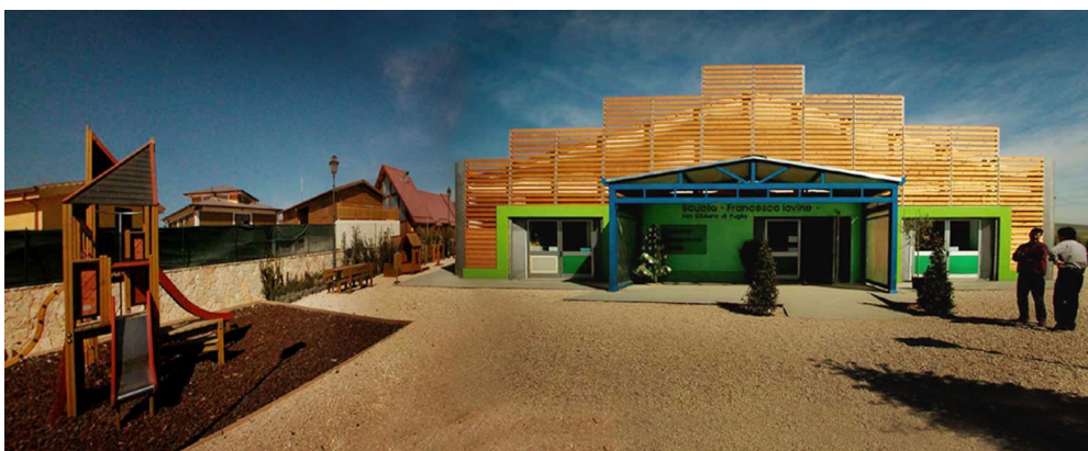
Figure 12. The new village temporary school has a simple wood slat “false front” to hide the prefabricated industrial profile of the building (Langenbach).
