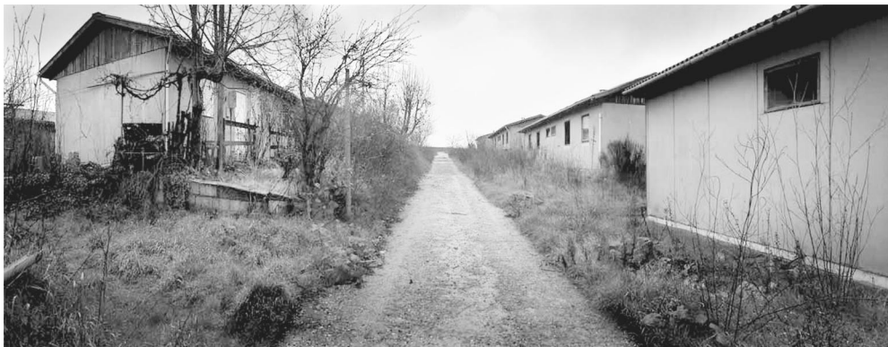
Figure 10. Calitri, in Campania. Demolition has been delayed because of the problem of safely removing and disposing of the asbestos cladding (Langenbach).
