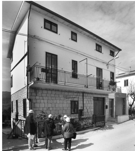
Figure 4. An inspection team meeting with the displaced owners of this dwelling prior to conducting a damage assessment of the interior (Langenbach).
