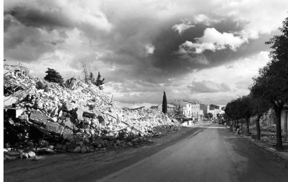
Figure 6. Demolition debris in the center of the expansion area of San Giuliano remained piled here for many months (Langenbach).
