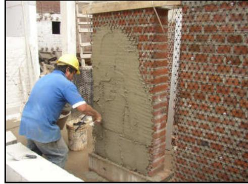
**Figure 5.** Plastering the panel.
