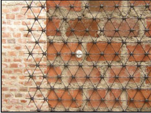
**Figure 4.** Polymer grid on panel.
